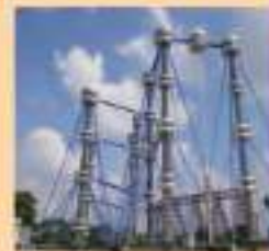
HVDC Generator at UHVDC, Hyderabad
