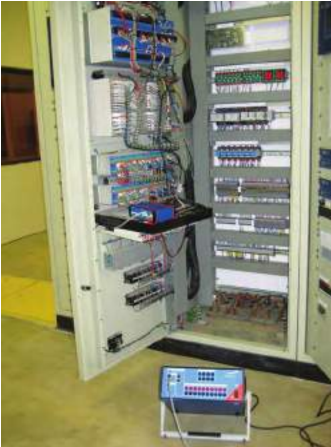
Figure 2: The DANE0 400 and the ISIO 200 can easily be connected to the communications network of substations in just a few steps.
