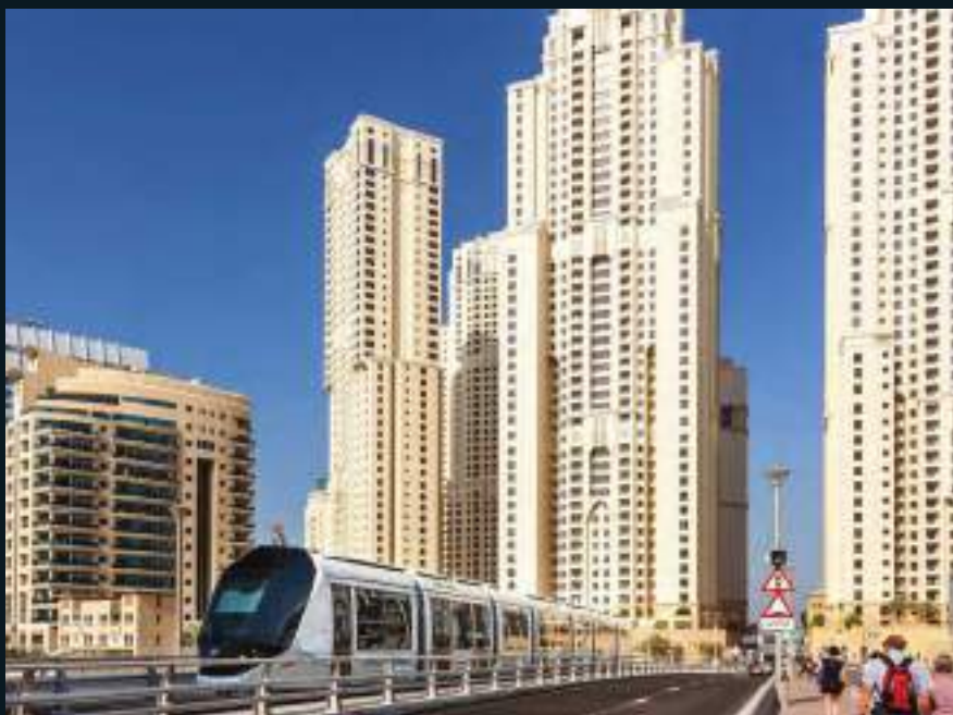
Fila provided products for use on the construction of the Dubai Tram. (Photo: Tatsiana Amelina)
