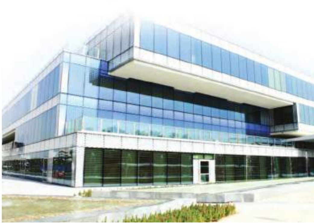
Al Jalilah Children Hospital in Dubai, which GEZE furnished with innovative technologies for automatic swing and sliding doors at the entrance and interior of the building.
