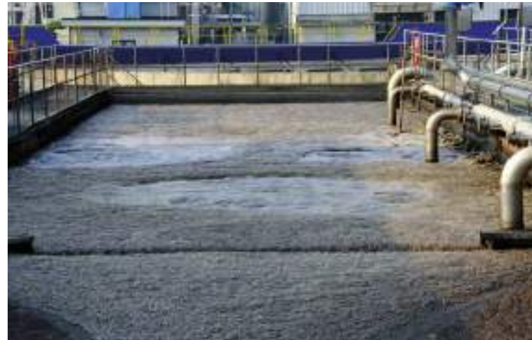
Sewage treatment plants can be made more acceptable by reducing the stench they produce. (Photo: Matteo Festi/Shutterstock)
