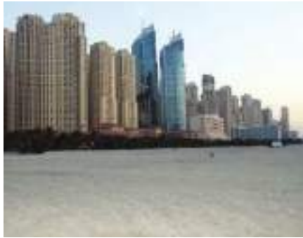
The environment in Middle East is highly corrosive with saline water and airborne salt damaging building near water bodies. (Photo: Imre Solt/Wikimedia Commons)
