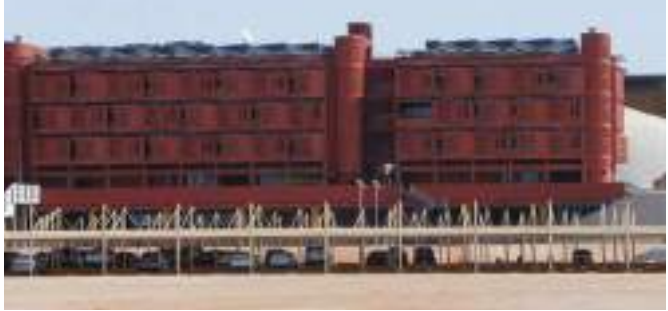
A number of projects throughout the GCC, such as Masdar City in Abu Dhabi, have helped raise the profile of 'green building' techniques. (Photo: Masdar)
